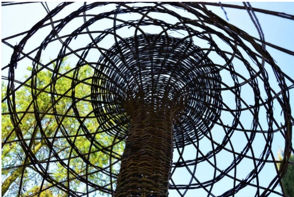
Figure 10: Willow kagome structure from below.
