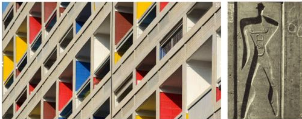
Figure 9: At Unité d'Habitation, in Marseille, Le Corbusier disposed of arbitrary metric measurements and replaced them with the 'remarkable resources of numbers' derived from his Modulor man.
