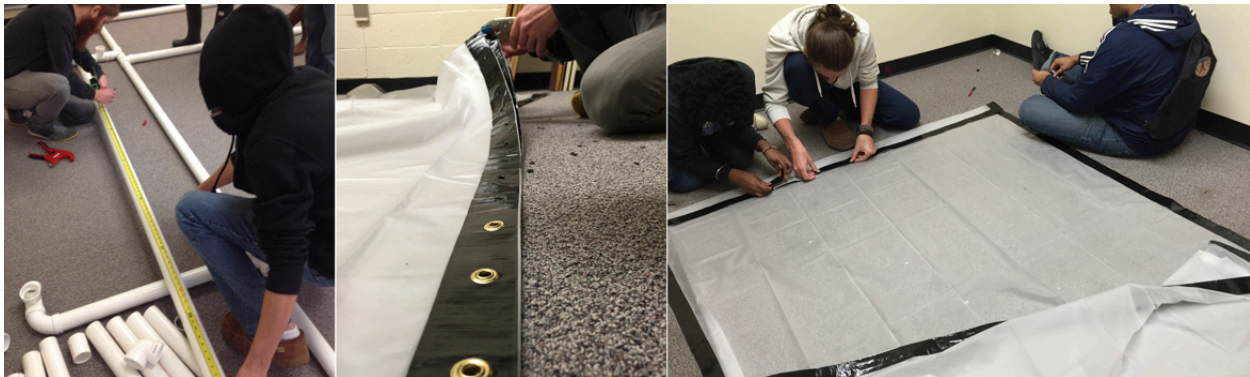
Figure 2: Students at the GameLab constructing CAVE structure using PVC pipes and shower curtain.
