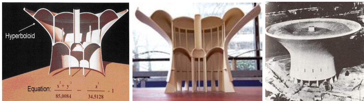
Figure 5: Water Deposit in Fedala (Eduardo Torroja, 1956). Project, scale model and real structure calculated with the geometry of a hyperboloid of equation (x^2 + y^2)/85.0084 - z^2/34.5128 = 1 .
