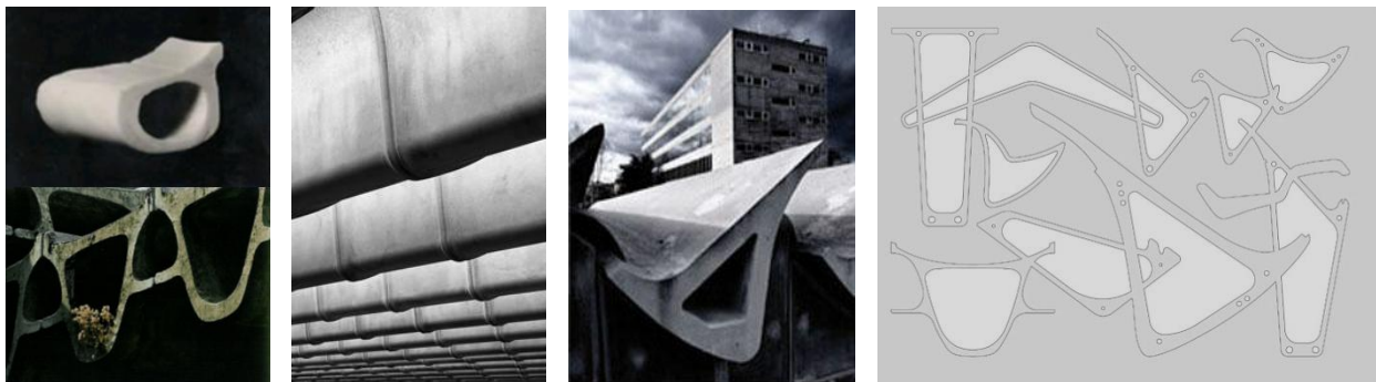
Figure 10: Miguel Fisac's "beam-bones". Inspired on real bones (top left) they integrate lightweight structures with beautiful designs.
