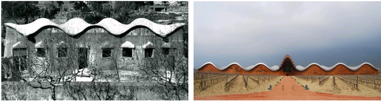
Figure 2: On the left, Escuelas de la Sagrada Familia (1909). On the right, Bodegas Ysios, Laguardia, (2001). Calatrava uses in the impressive winery Bodegas Ysios the same geometry based on conoids that Gaudí used on his small School at the Sagrada Familia in Barcelona.
