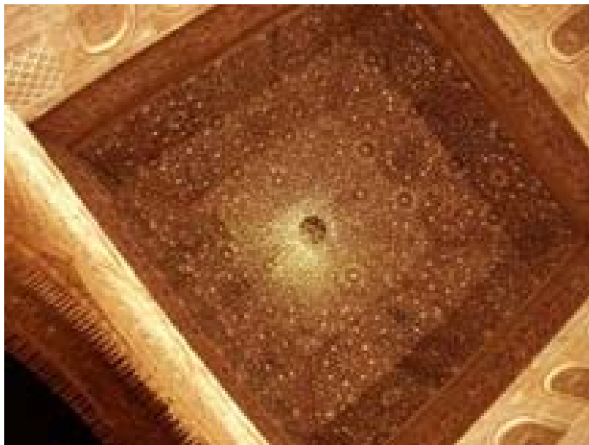
Figure 4: View of the Seven Heavens ceiling
