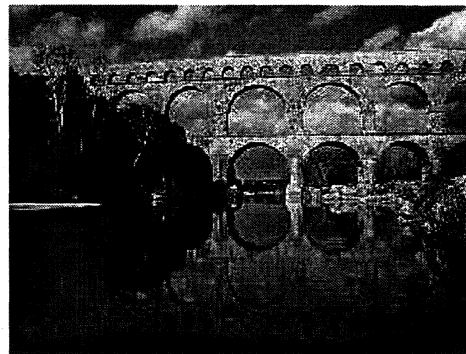
Figure 11: Roman aqueduct (20 B.C.) (Nimes, France)
